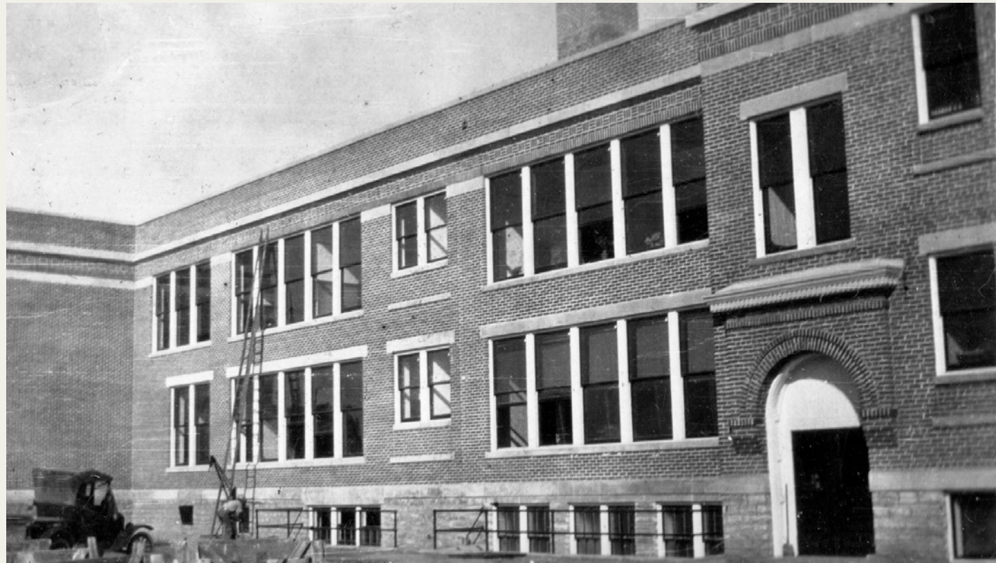
Historic image of the Spring Grove Public School under construction
